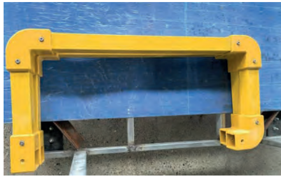
Fig. 3.5: Image of top handrail with bolts
