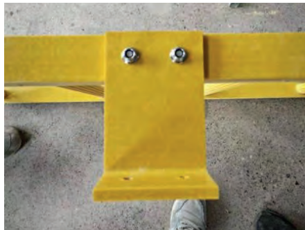
Fig. 3.2: Assembly of wall brackets
